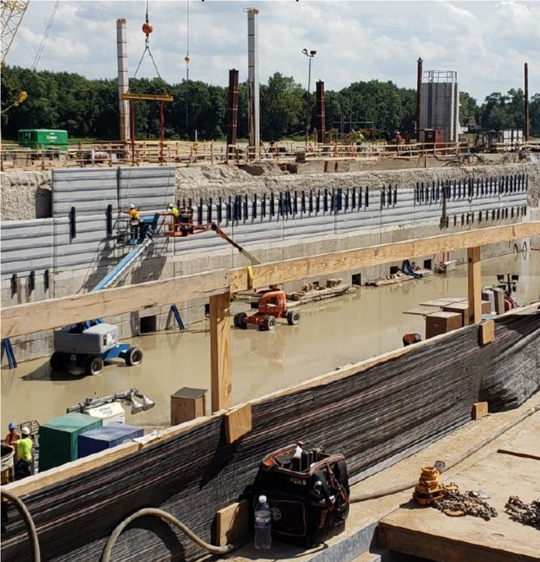
Vertical concrete pre-cast panel installation
